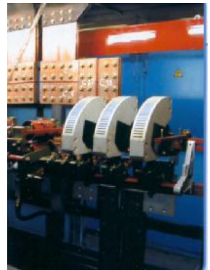
Type: CBA 98 4500A 2.0 Operating voltage: 3500Vac, Ith : 4500A Breaking current @ \cos \varphi = 0, I : 25 \text{ kA}
